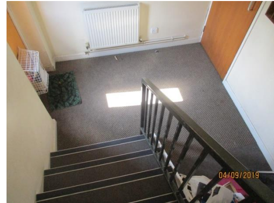
Photograph (6)- General view of the ground floor access landings
