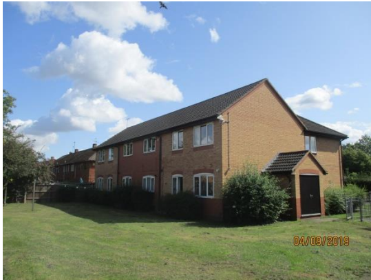
Photograph (21)- Rear elevation of Block 1-6
