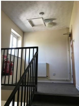
Photograph (7)-General view of the upper floor access landings
