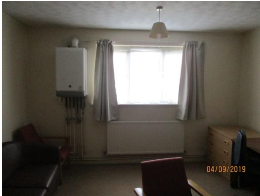
Photograph (5)- Typical sitting room to the flats
