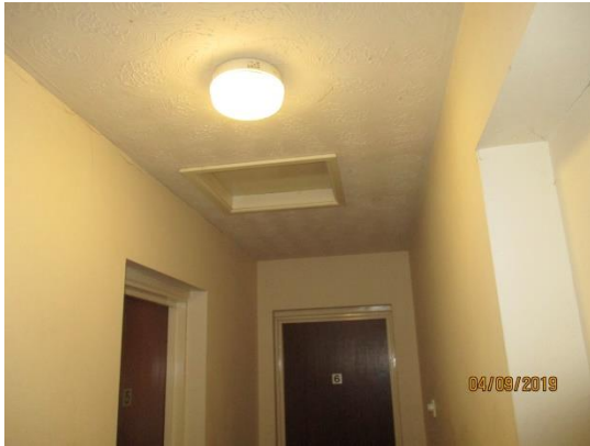
Photograph (17) - General view of the upper floor hallway to Block 1-6
